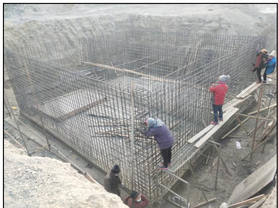
渗滤液池绑钢筋
